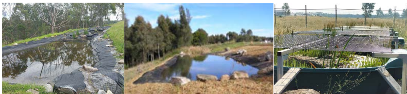
Figure 8. Examples of some of the wetland types successfully used at the Sydney Olympic Park for the Green and Golden Bell Frog L-R: Plastic Tarp lined breeding ponds; Rubber HDPE lined pond; Plastic trough (now installed by the City of Whittlesea in Epping).
