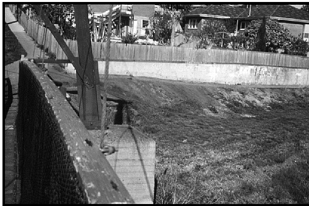
Kendall Street footbridge in Preston.
